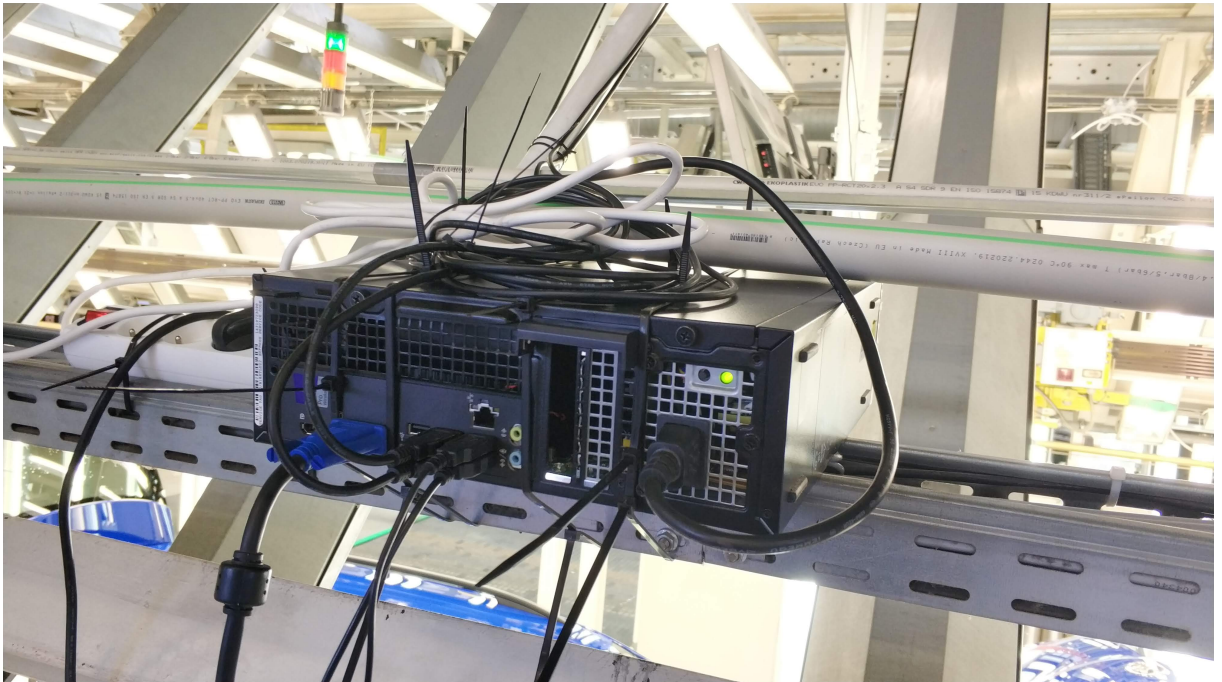
Figure 2.2: Computer was also attached to the construction above the conveyor.
